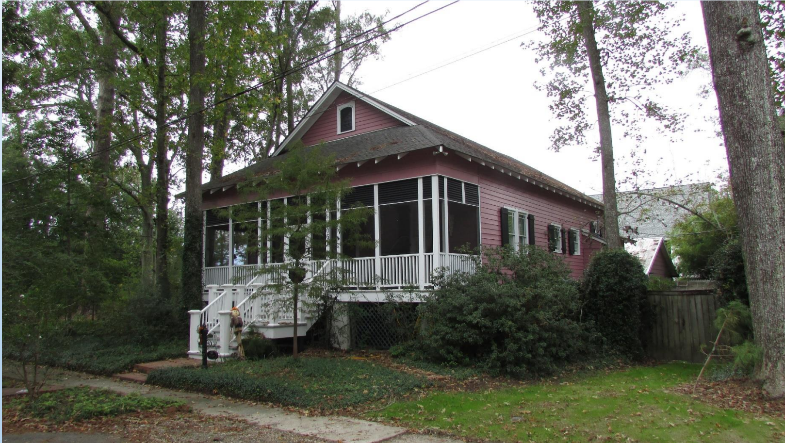
LOW ELEVATION WITH OPEN FOUNDATION
