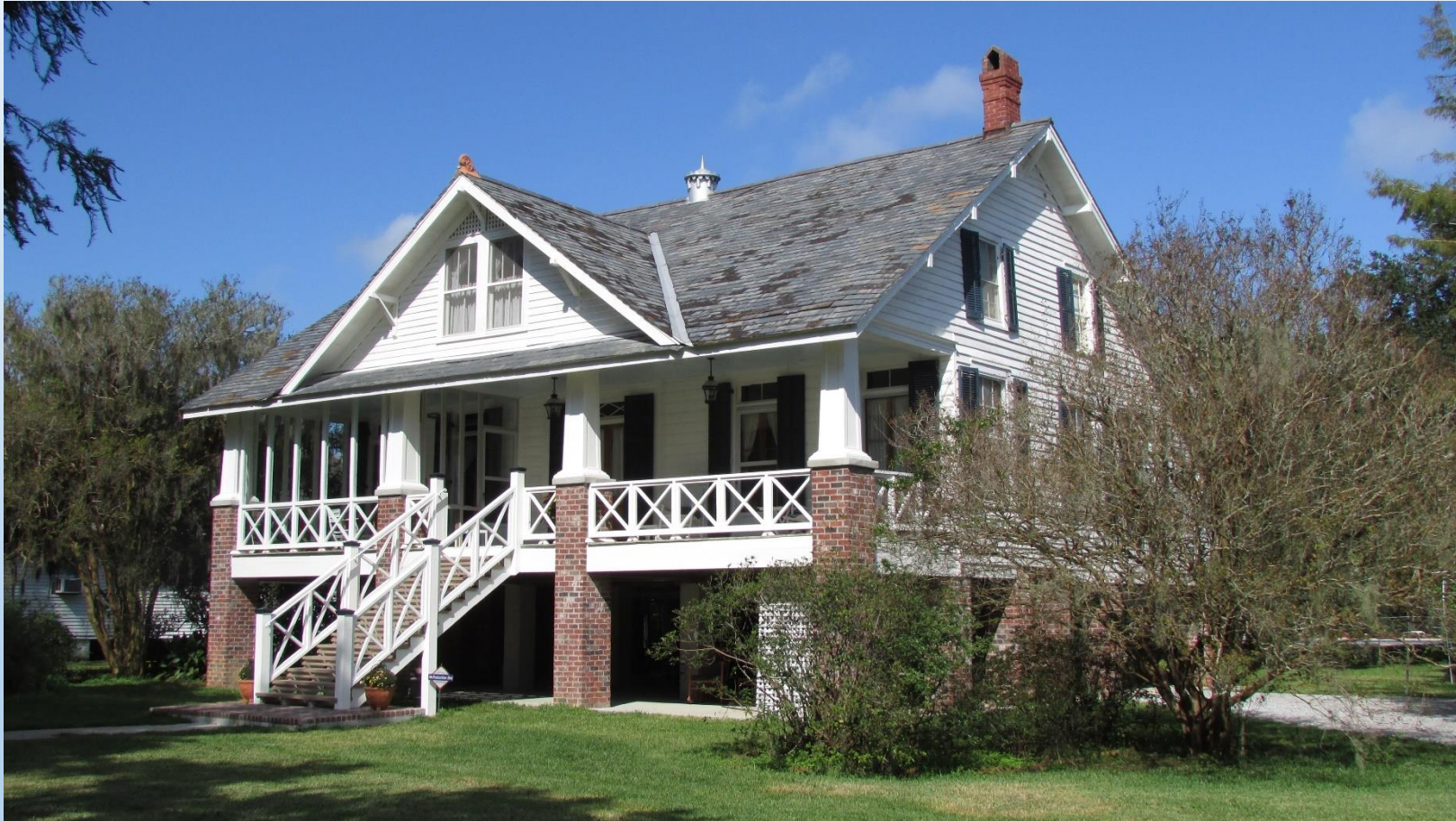
HIGH ELEVATION OPEN FOUNDATION
