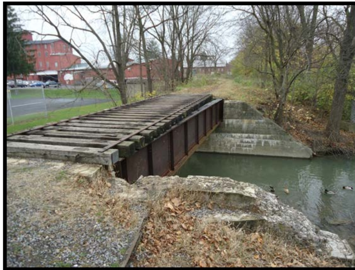
Figure 7.8 - Small Steel Girder Bridge over Bull Run
