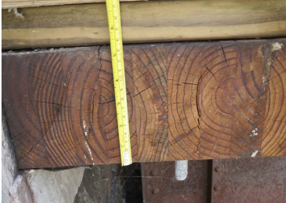
Figure 7.13 Glulam Deck Panel Orientation
