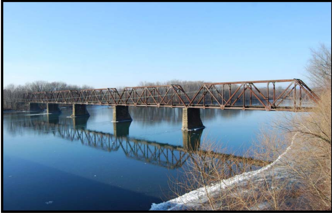
Figure 5.2 - Railroad bridge over the Susquehanna River. (Alexander Mitchell IV, 2010)
