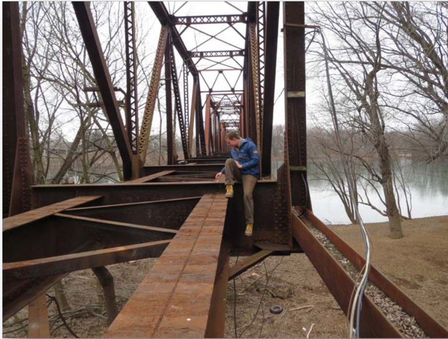
Figure 7.15 - Team Members measuring size of steel members
