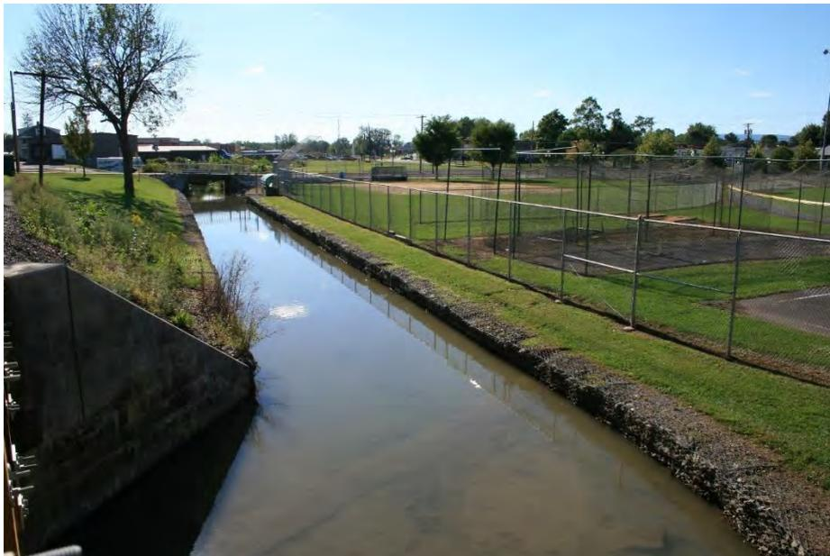
*The Bull Run stream that flows through Daniel Green Park is lined with rock gabion cages to provide streambank stability. This reach of stream has little slope and suffers from a build-up of sediment in the stream channel.*
