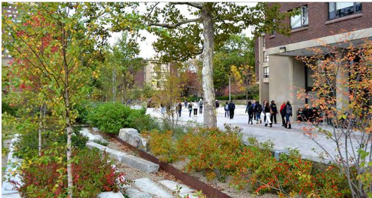
'Artful' Stormwater Management – a different approach will be taken handling stormwater runoff from the street and sidewalk. Lack of curbing on the east side of street will allow water to sheet flow and be captured in runnels, rock splash feature, and wetlands, treating the water before it is discharged into Bull Run.
